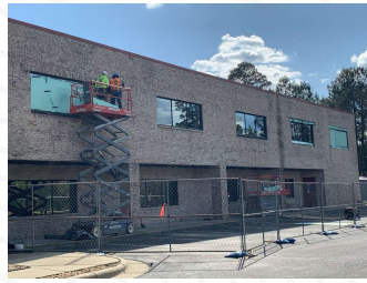
NORTH-SIDE WINDOW REMOVAL, SECOND FLOOR
