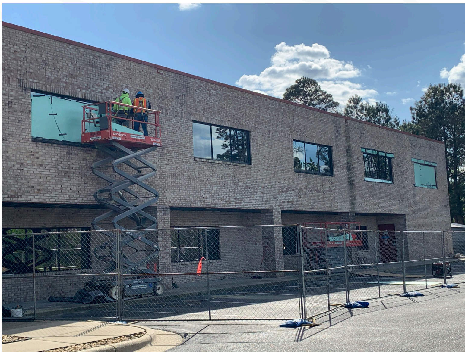
NORTH-SIDE WINDOW REMOVAL, SECOND FLOOR
