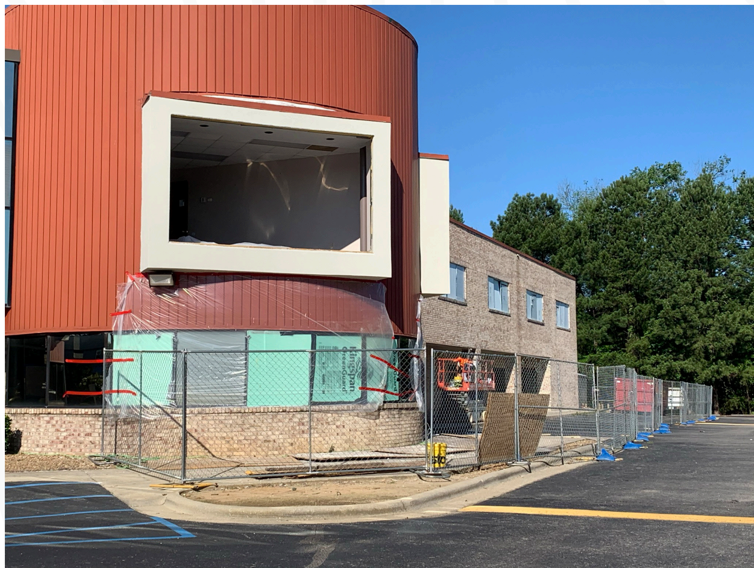
RIGHT ROUND WINDOW INITIAL SQUARING FOR REPAIRS
