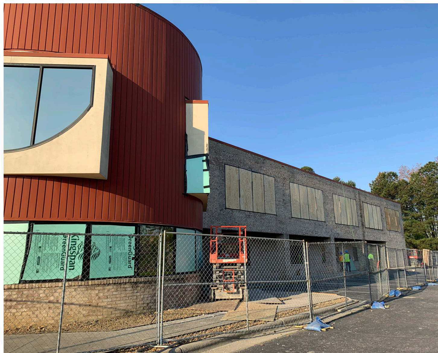
NORTH SIDE WINDOWS ENTIRELY REMOVED, SECOND FLOOR
